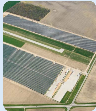
Partial aerial view of PSEG's Wyandot Solar facility. The panels cover approximately 80 acres.
